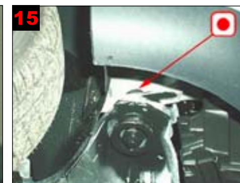
15 Longitudinal member front: Treat via existing plugged hole.
